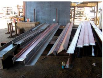
Figure 3-10. Steel Beams Coated by Architectural Contractor
