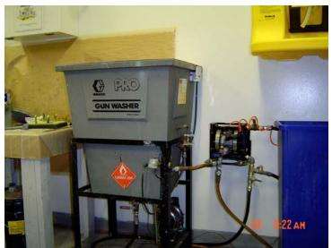
Figure 3-9. Typical Spray Gun Cleaning System
